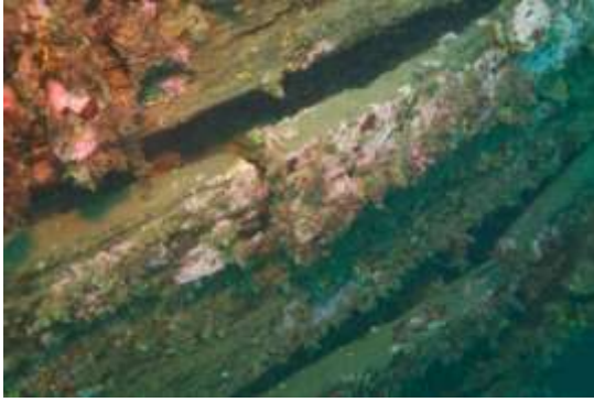
Fig. 6: In many areas hull planks have started to loosen due to the internal pressure and the oxidation of the iron bolts (N. Mouchart).
