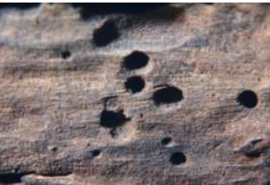
Fig. 9: Close up of bore holes wood boring mollusca such as the Teredo Navalis (N. Mouchart).
